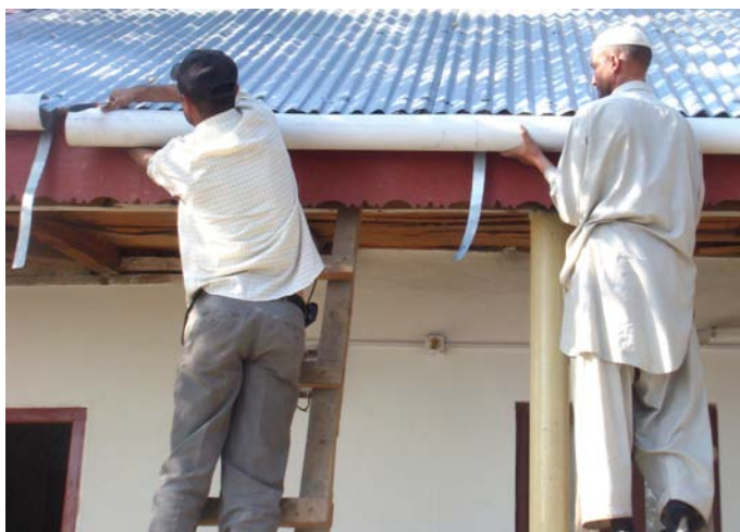
Installation of rainwater harvesting system pipes, photographed by CWS-P/A staff
